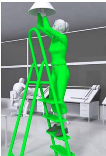
Example where two hands need to be free for a brief period for light work. Keep two feet on the same step and the body (knees or chest) supported by the stepladder to maintain three points of contact. Make sure a safe handhold is available
